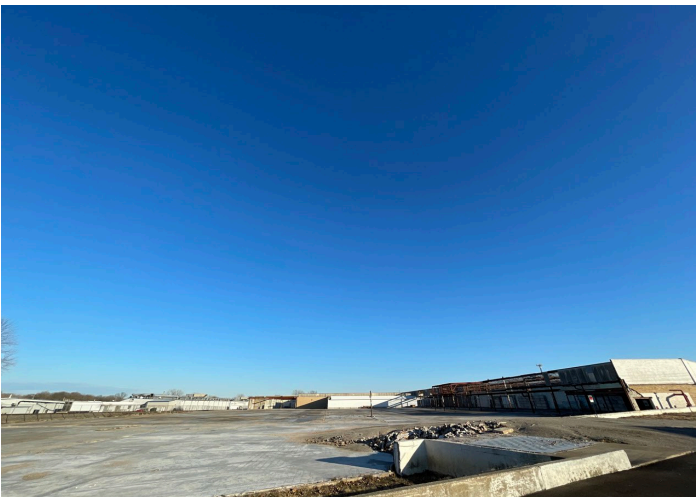
Deteriorated structure at Industrial site on S. Dickey Street.
