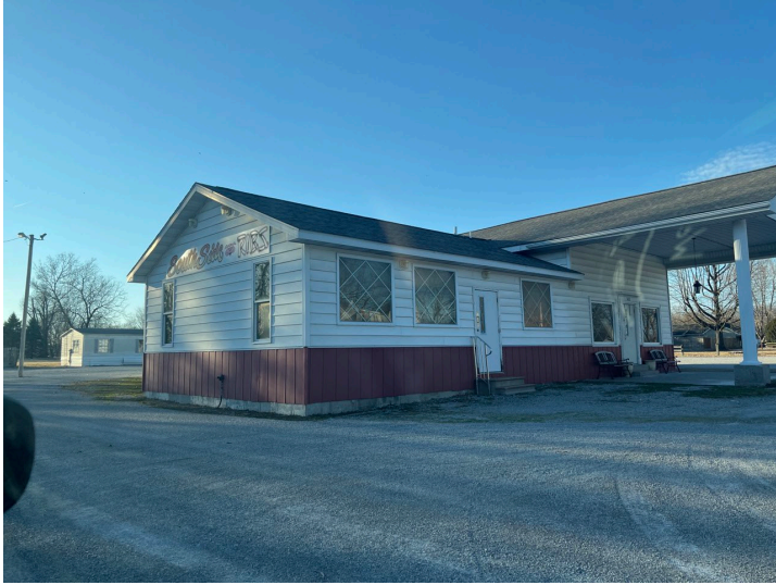
Deteriorated parking area at 903 S. St. Louis Street.
