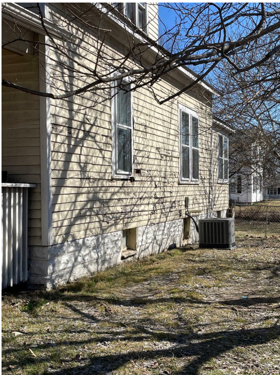
Dilapidated structure at 514 S. St. Louis Street shows signs of buckling exterior walls, deteriorated windows and siding.
