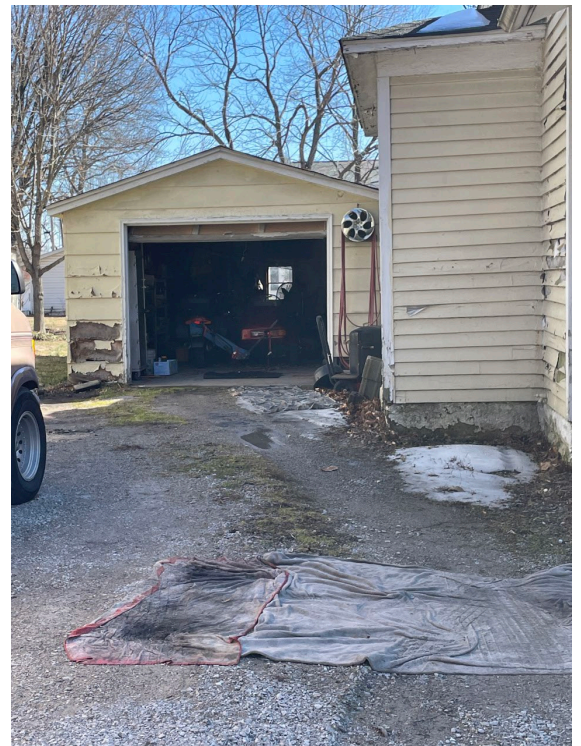
Dilapidated structure at 514 S. St. Louis Street shows signs of buckling exterior walls, deteriorated windows and siding.
